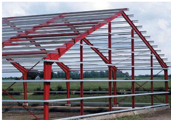
Building with hot rolled frame and cold rolled Z-purlins
